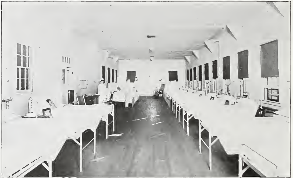
FIG. 126.—A ward, Post Hospital, Eberts Field, Ark.
